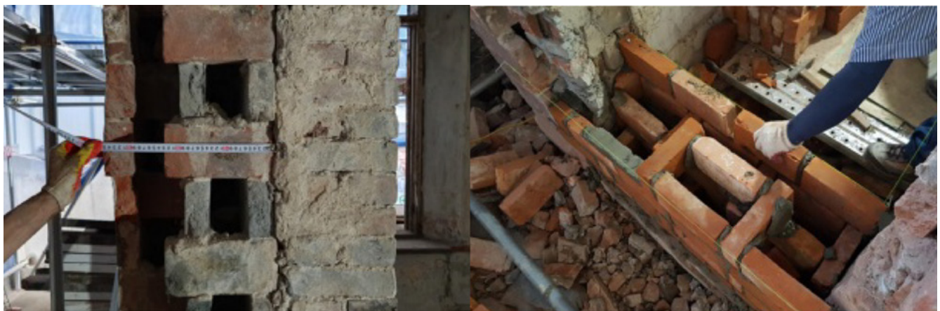
Photo 3.8 Conservation works of Rat Trap bond to maintain insulation function and structural stability
