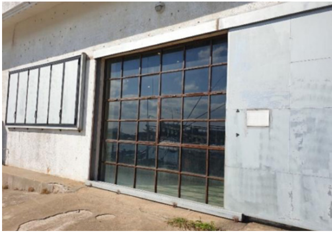
Photo 5.7 Energy-saving insulation glass and natural light employed for inside lighting
