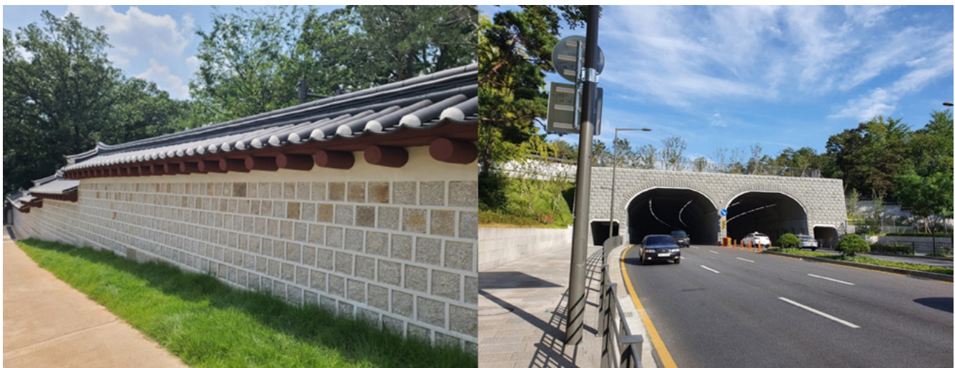
Photo 3.12 Adaptation approach: Changdeok Palace walls, reconstructed using more than 20% of the stones excavated during the restoration, and six-lane concrete tunnel for vehicular traffic
