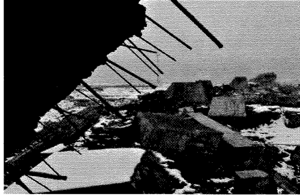
Figure 10-2. Super bank destroyed by Tsunami 2011 super bank destroyed by Tsunami 2011 at Taro, Miyako City: Sankei News , March 16, 2011 http://yoiotoko.way-nifty.com/blog/2011/03/post-f16e.html
