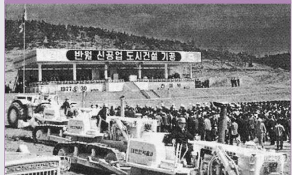
Banweol Industrial Complex Groundbreaking (1977)
