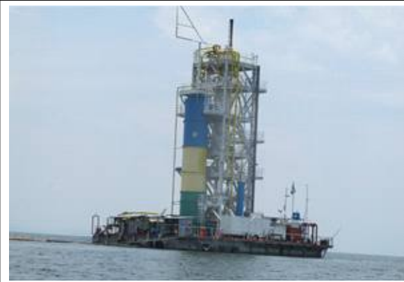
< Kivu Power Generation >
