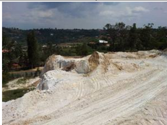
< Local Housing Construction Site -2 >
