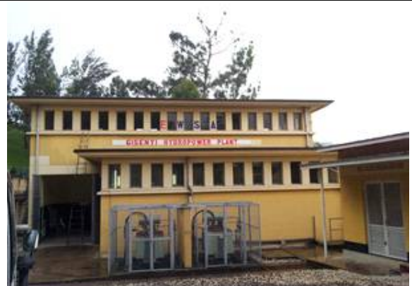
< Gisenyi Hydropower Plant >
