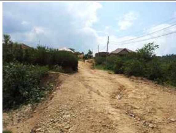
< Local Housing Construction Site -1 >
