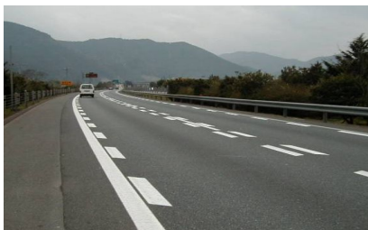
Channelizing Lane Marking
