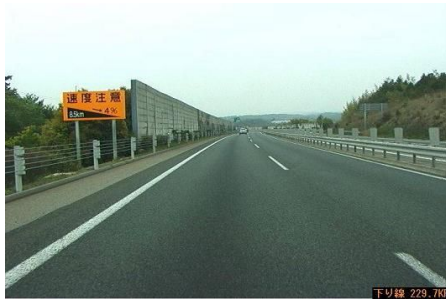
Attention Causing Sign in Downward Section
